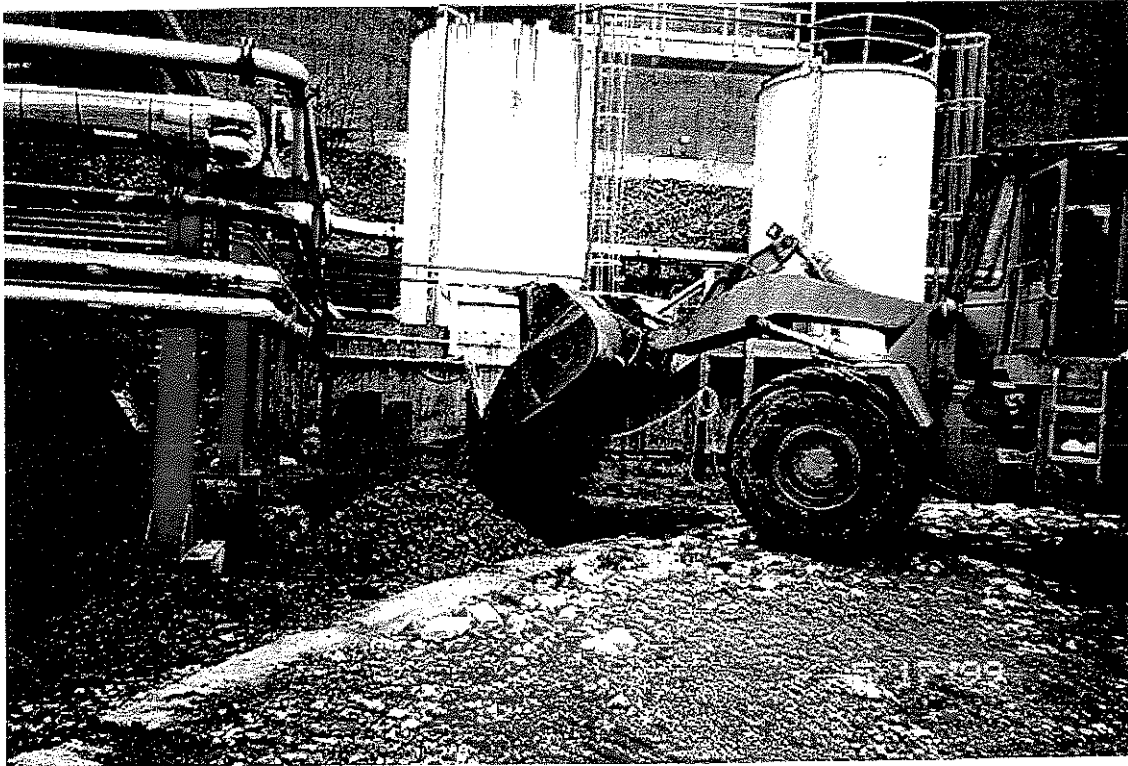
Photograph 1. Backfilling of excavation area between foundation ring and containment berm, May 1999.
