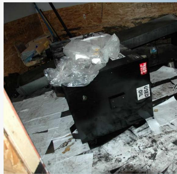
Used oil container toppled during flood; it could be elevated and anchored.
